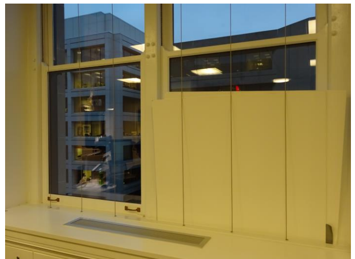
An occupant installed an additional foam core board, clearly dissatisfied with amount of shading from automated mesh shades.
