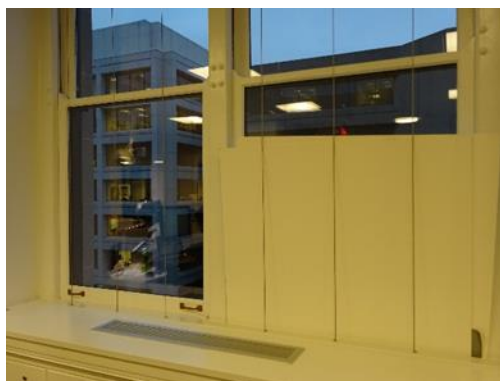
Figure 9. To reduce window glare more effectively than mesh window shades, an occupant installed an additional opaque board.
