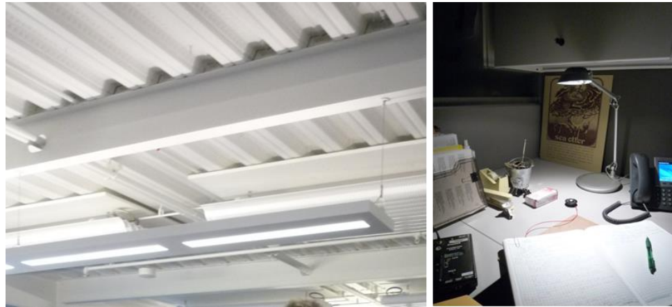
Figure 3. Typical luminaires in open office areas.
