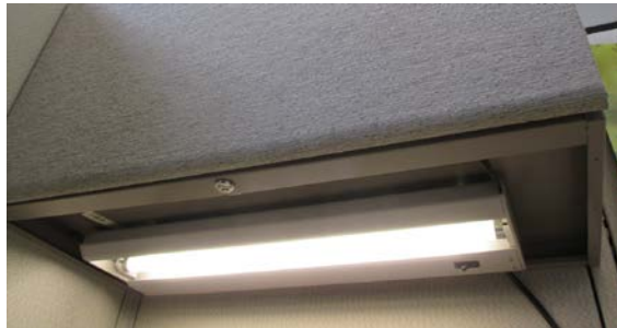
Figure 3. Task lighting is available at desks on the first floor.
