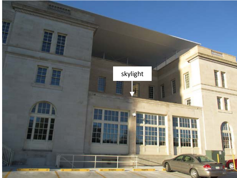
Figure 4. On early summer mornings, some direct sun falls on the north side of the building. The skylight on the first floor is well-shaded on this north side of building.
