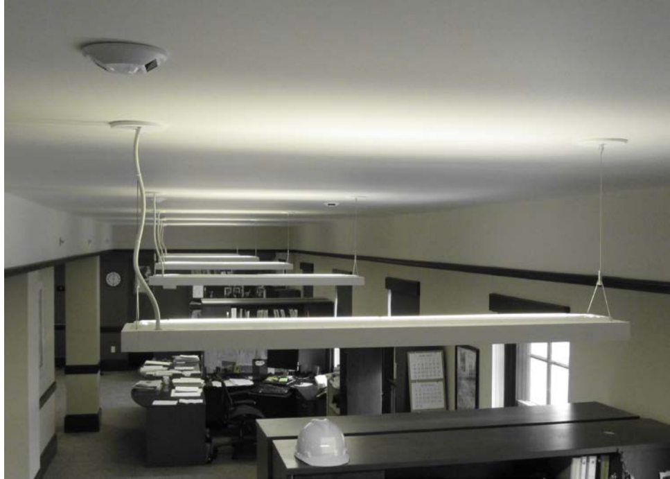
Figure 2. Linear fluorescent pendants provide the general lighting in open-plan offices. Wireless sensors (upper left) help to reduce energy use by dimming the lights in response to daylight and switching them off when the offices are vacant.
