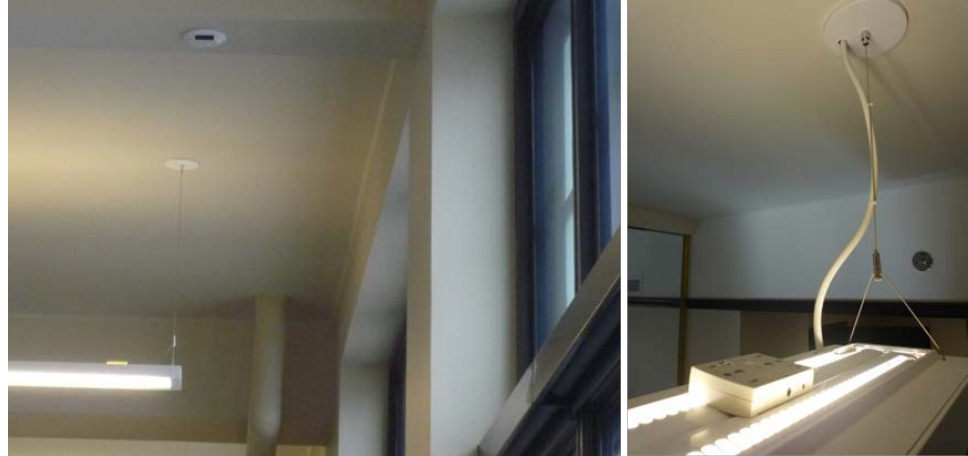
Figure 13. (A, left) Battery-powered light meters were installed in two locations on the first floor, and one location on the second floor. (B, right) A close-up of the sensor measuring light passing through uplight slots.
