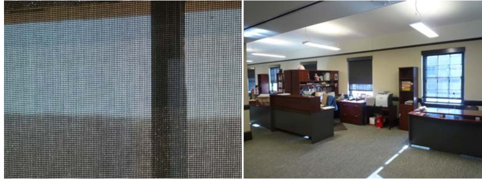
Figure 4. (A) A close-up of the translucent black mesh shades personnel with south-facing windows have the option to use. (B) Although one window has blackout shades retracted, the sun may not be “seen” by the photosensors in the room.
