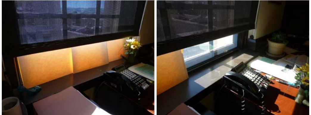
Figure 7. (A, left) As the mesh shades on this second floor south window are not long enough to fully cover the window, the occupant of this desk uses office supplies to shield the sun in the winter. (B, right) The sun hits the desk through the gap between the shade and window when the window is not covered.
