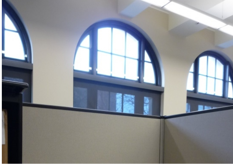
Figure 2. West-facing windows are fitted with black mesh shades.
