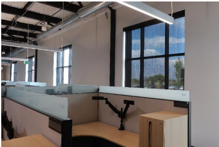
Figure 17. Mesh window shades kept closed for reasons of glare and privacy concerns; closed mesh shades do provide view to exterior.
