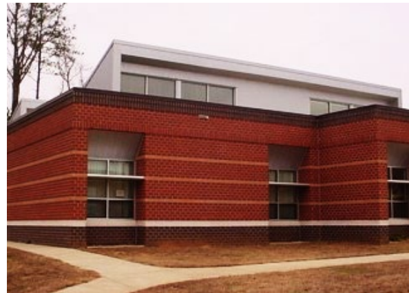
Figure 2. This school building employs south-facing roof monitors and deep-set windows with light shelves to provide daylight to classrooms but limit glare from direct sunlight.
