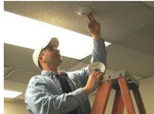
Figure 8. A commissioning agent makes adjustments to a lighting control device.
