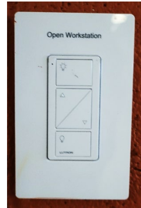
Figure 10: A manual lighting control in an office allows workers to adjust light levels.
