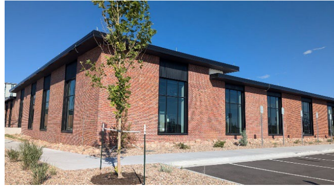
Figure 7. Plantings near the windows of this office building are kept low so as not to block daylight into the interior and light-colored groundcover is used near windows, which reflects daylight.
