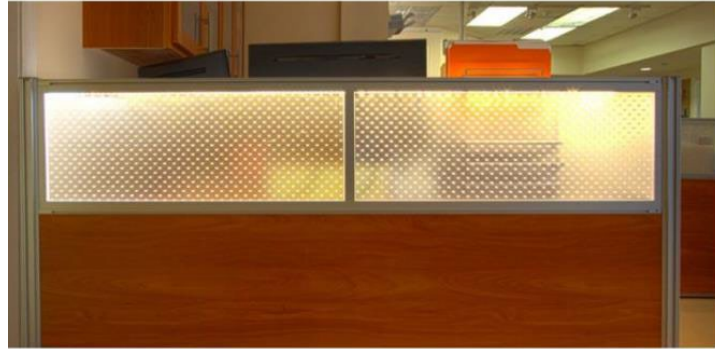
Figure 6. An example of circadian-effective light integrated into a cubicle in an open plan office.
