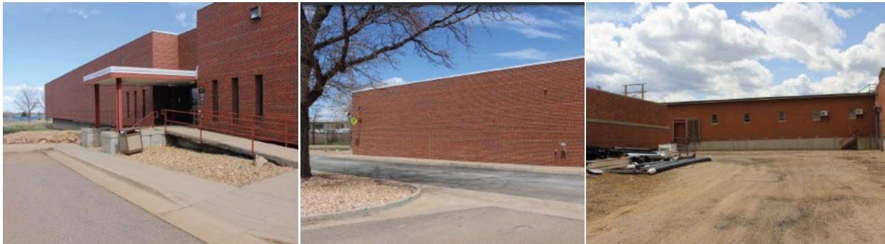
Figure 1. Exterior pictures of Building 48 on the DFC campus in Lakewood, CO prior to renovations.
