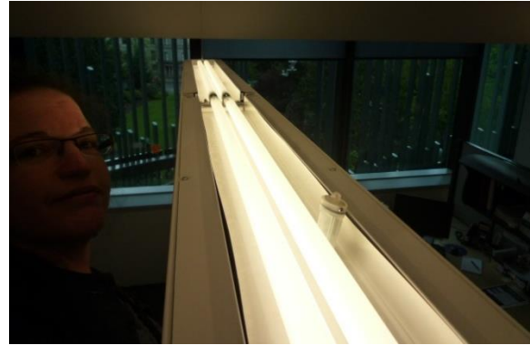
Figure 15. LRC researcher installs a battery-powered light meter in a luminaire at EGWW.
