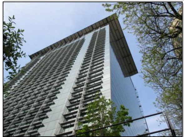
Figure 1. EGWW is a newly-remodeled, high-rise office building with “reeds” on its west side (center) and other exterior shading devices on the south and east sides (lower).
