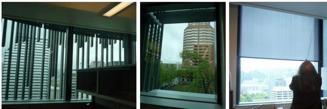
Figure 6. As seen from inside, architectural “reeds” provide exterior shading on the west side of the building (left), while other exterior shading devices are used on the south and east sides (center). Adjustable mesh shades are also provided (right).
