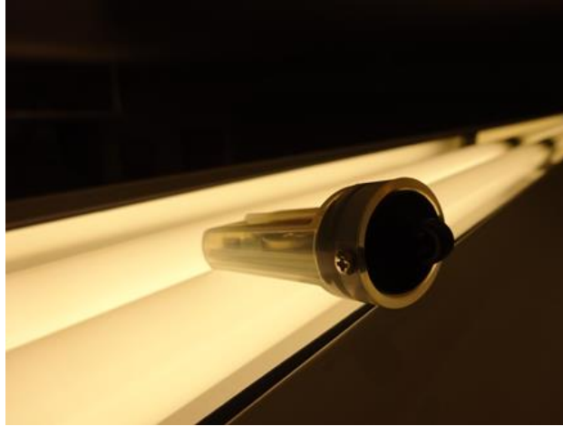
Figure 8. Battery-powered light meter in a luminaire during winter evaluation.
