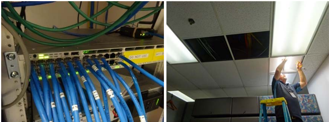
Figure 9. Electrician connected each light to the dedicated Cisco server (left); as shown on the right, the luminaires could easily be moved from one location to another. Also shown at right, the two luminaires have not yet been programmed to match color temperature.
