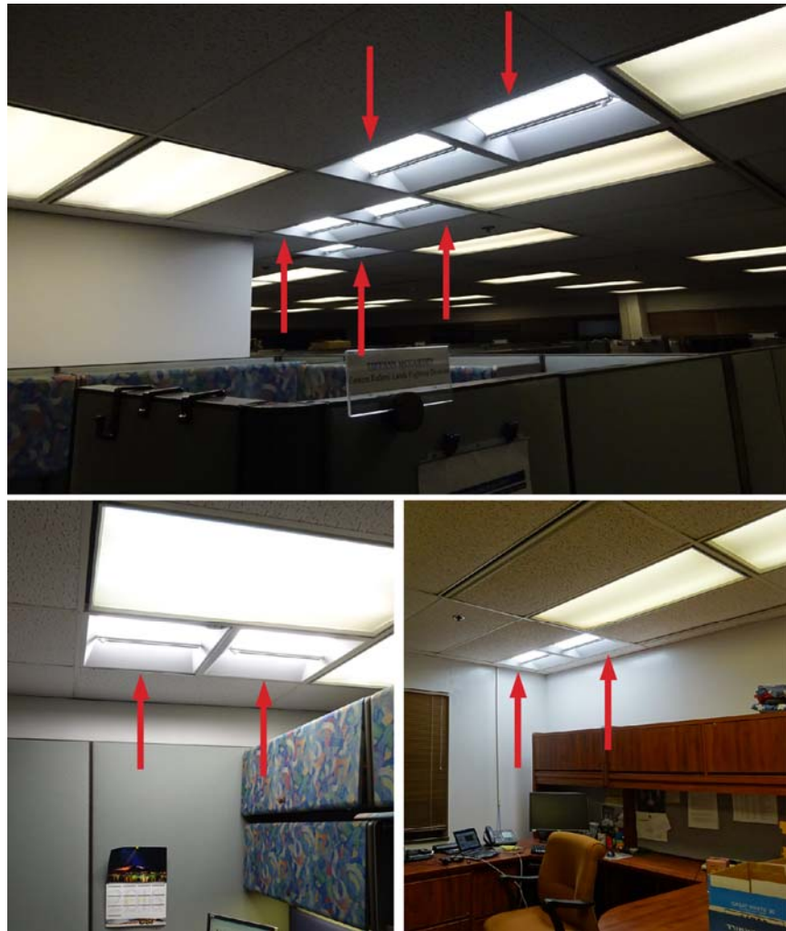
Figure 10. Examples of CREE 2x2 troffers (indicated by red arrows) used as lighting intervention at the FHWA site.
